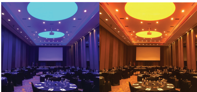
RGB LED Fixture (making full use of 4-channel output)
